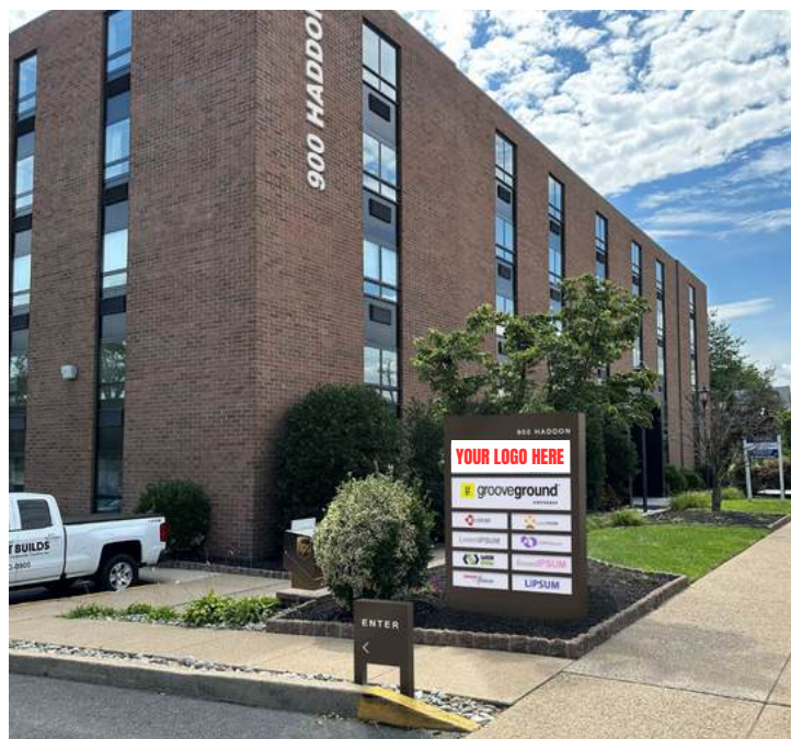
EXTERIOR DIRECTORY SIGNAGE
